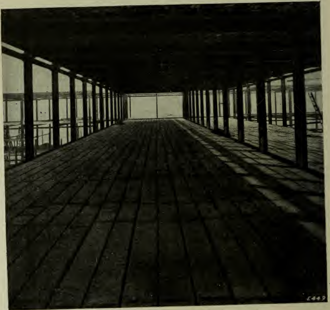
THE NEW PENSIONS BUILDING, ACTON: FLOORS DURING CONSTRUCTION.
